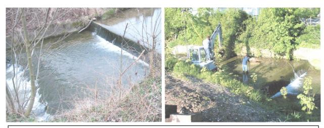
Weir built in the 1950s and representing an obstacle to fish migration in the river "Lauter". Initial state before the implementation of the compensation measure in 2008. (Source: StadtLandFluss, internal documents).
